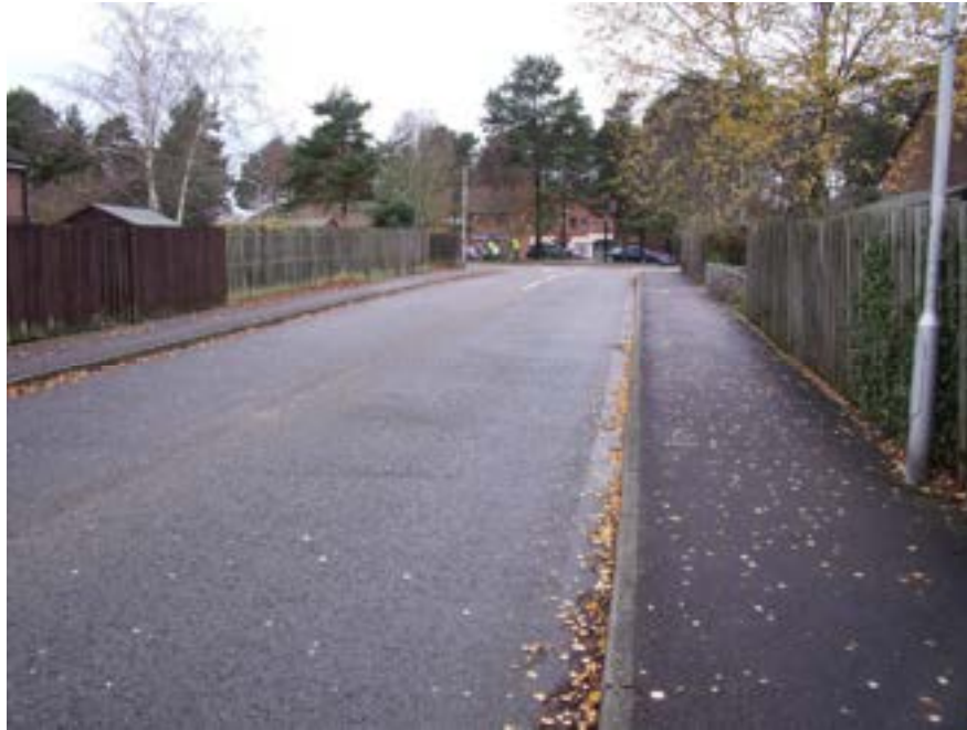
Photograph 3.10: Nuneaton looking west towards Opladen Way
