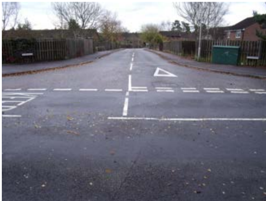
Photograph 3.11: Nuneaton looking east towards Bruton Way
